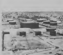
VIEW ON huge 630,000 bbls tank. VISTA RIBA tanki di 630,000 bariil.
